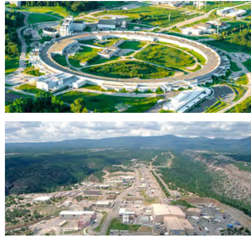
Figure 16: DOE user facilities, such as the Advanced Photon Source (top) and the Los Alamos Neutron Source Center (bottom), can enable the development of novel characterization tools to probe electronic materials under nonequilibrium conditions, such as high frequencies and fields, at extreme temperature and radiation environments.
