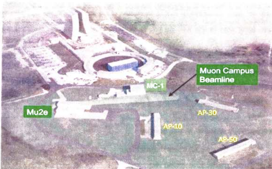
Figure 2 The Fermilab Muon Campus including the Mu2e Facility, the MC-1 Building, the Muon Campus Beamline berm, and the former Antiproton Facility Buildings (AP-30, AP-10, and AP-50)
