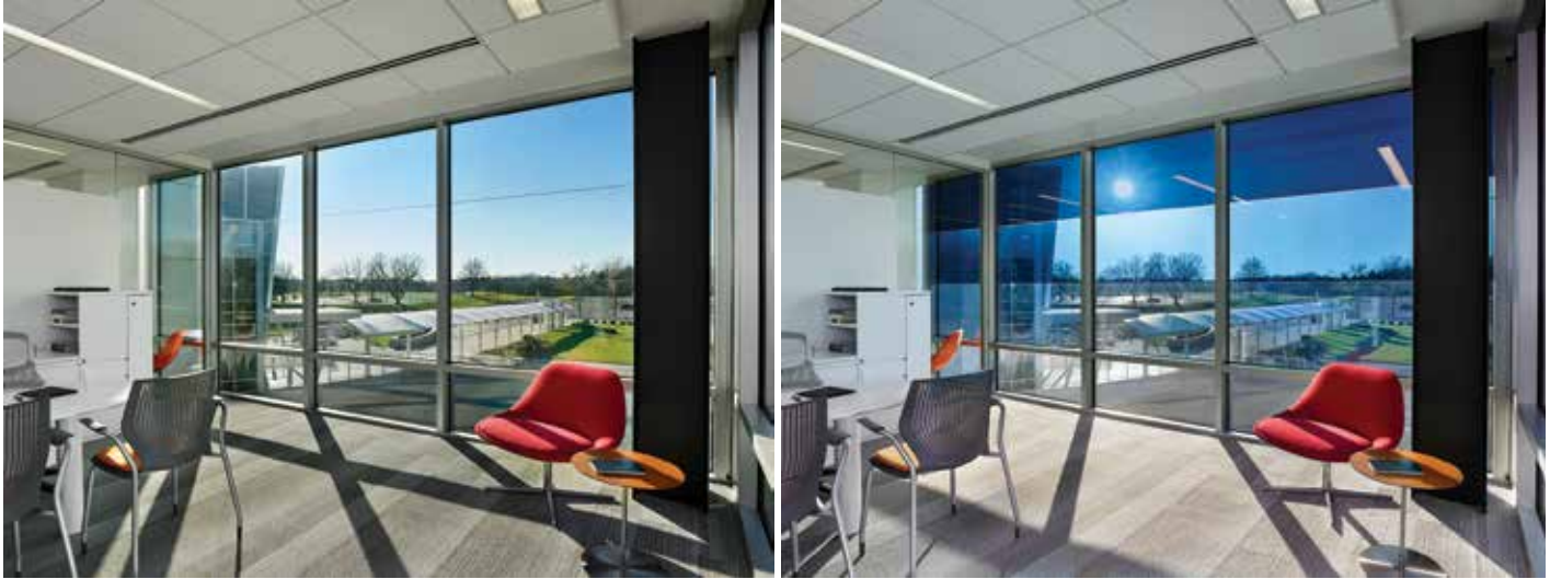
These “smart” windows make use of specialized materials to change their tint and lower the amount of sunlight transmitted in response to environmental conditions, saving energy for cooling buildings and creating more comfortable working conditions. ( SageGlass, Inc )
