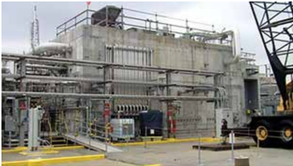
Modular unit nearing completion at the Savannah River Site for removal of radioactive cesium using the chemistry developed at Oak Ridge National Laboratory. (U.S. DOE Savannah River Site)
