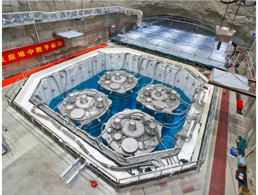
Daya Bay Far Detector Hall with 4 neutrino detectors
