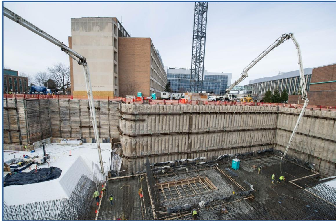
Concrete for the floor of the target area was placed December 1-2. It took around 30 hours and 300 concrete trucks to place the 2,700 cubic yards of concrete. FRIB received Critical Decision 3B, Approval to Start Technical Construction, on August 26, 2014.
