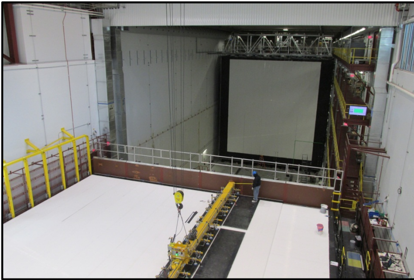
Workers at the NOvA hall assemble the final block of the far detector in early February 2014, with the nearly completed detector in the background. Each block of the detector measures about 50 feet by 50 feet by 6 feet and is made up of 384 plastic PVC modules, assembled flat on a massive pivoting machine.
