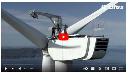
Figure 8: A self-hoisting crane demonstration Click <u>here</u> to see video
