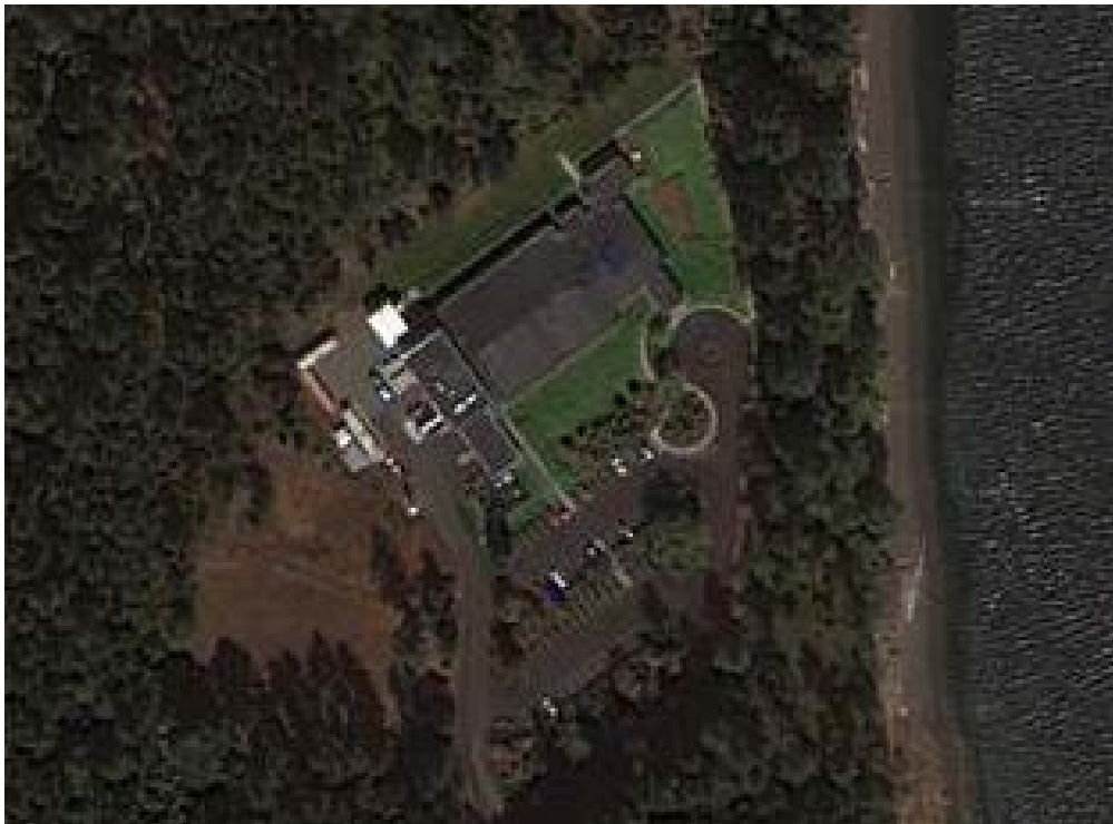
Figure 1.4. Overhead View of Building MSL-5
