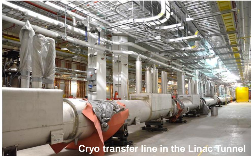
Cryo transfer line in the Linac Tunnel
