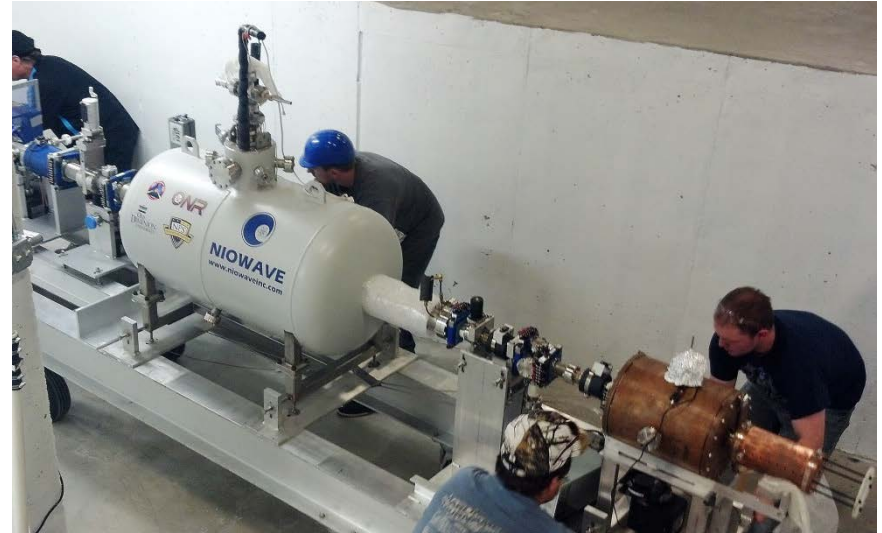
A superconducting linac being installed in a Niowave testing tunnel
