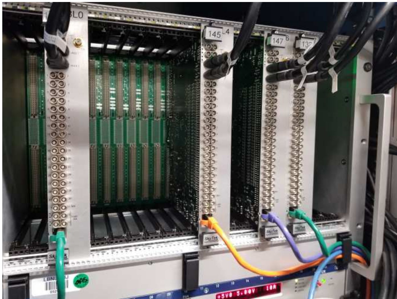
DDC-32 Boards being Installed in the SURF Lab Underground
