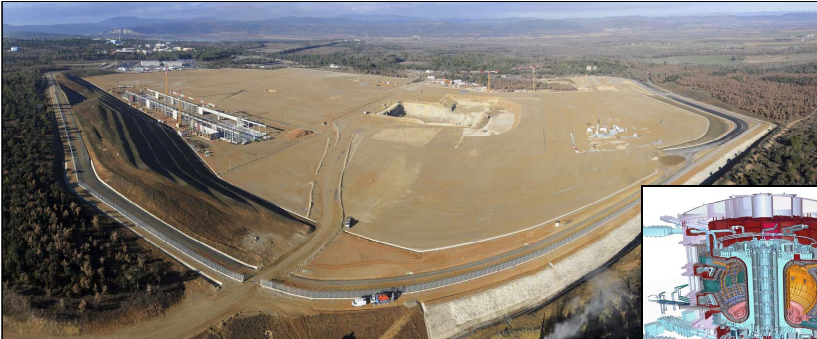
Site construction is underway in Cadarache, France
