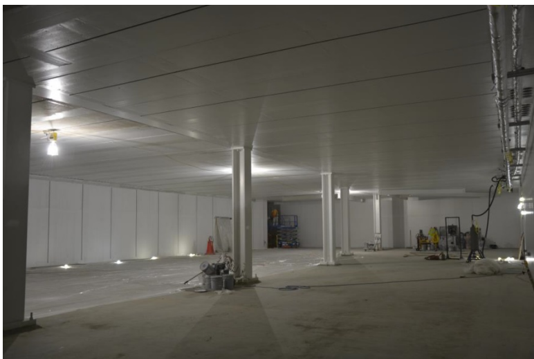
Tunnel warm and painted
