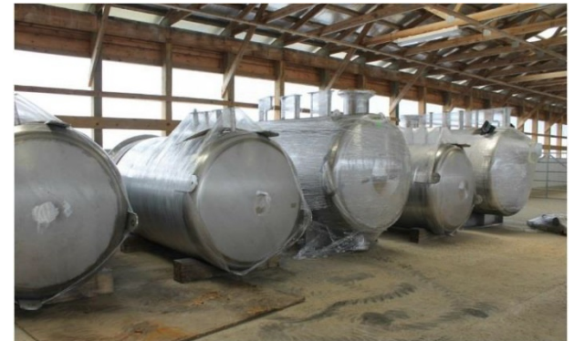
Five of fifteen nonconventional utility process tanks to be installed during conventional construction.
