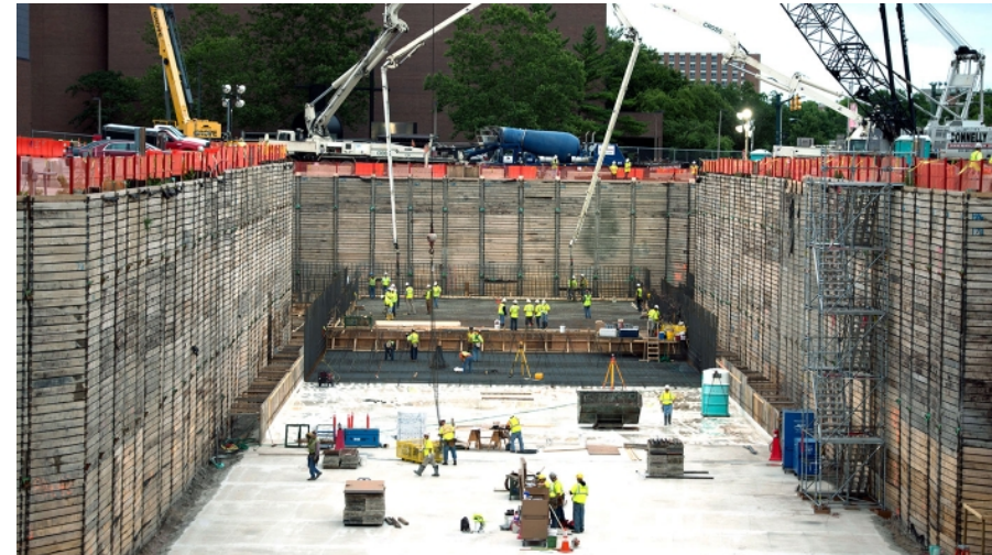
In July 2014, 140 truckloads of concrete arrived at MSU.
