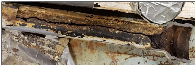
Spedding Hall Deteriorating Sewer Piping (circa 1953)
