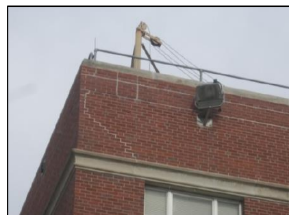
Spedding Hall Deteriorating Brick/Limestone Exterior (circa 1953)
