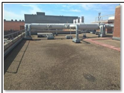
Spedding Hall Existing Built-Up Roof (circa 1985)
