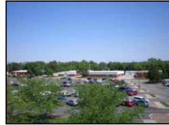
Shop Buildings and Warehouse (1964-1991)
