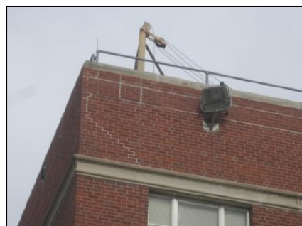
Spedding Hall Deteriorating Brick/Limestone Exterior (circa 1953)
