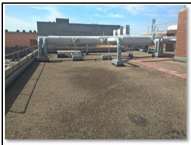
Spedding Hall Existing Built-Up Roof (circa 1985)
