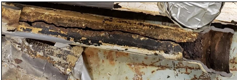
Spedding Hall Deteriorating Sewer Piping (circa 1953)
