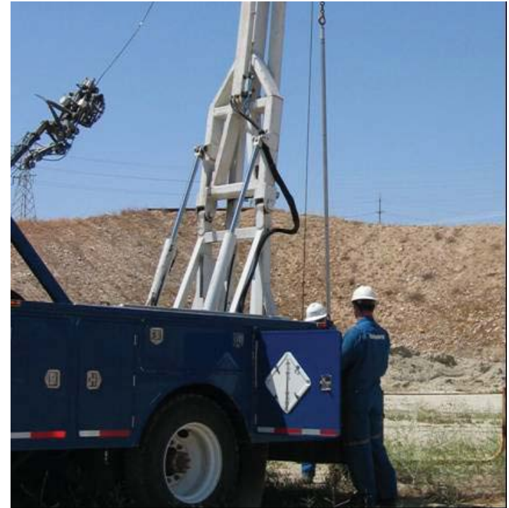
Workers preparing a small-diameter well probe that contains a neutron generator for use in logging an existing oil well borehole.
