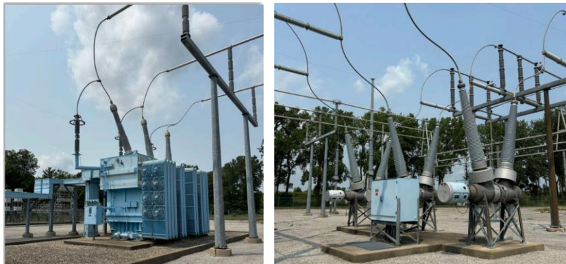
345kV Transformer and Circuit Breaker to be replaced
