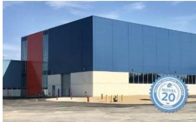
Industrial Center Building Addition received recognition as a new building that performs above code thanks to the design of its building envelope, which includes windows, exterior walls and roofs. In fact, its building envelope surpassed the award’s criteria of a 20% improvement over current building code, providing a 25% improvement.
