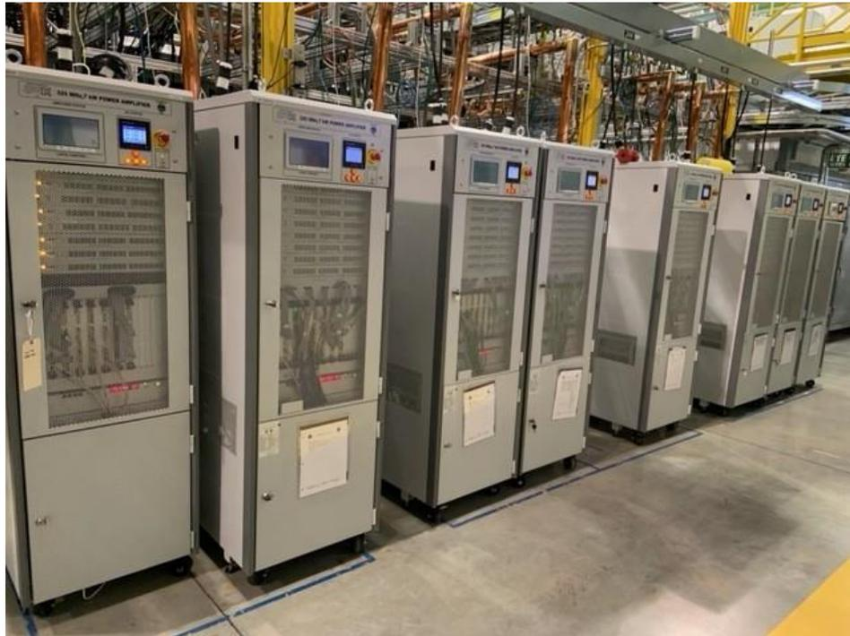
ECIL/BARC 7 kW 325 MHz amplifiers powered SSR1 cavities during beam testing at PIP2IT
