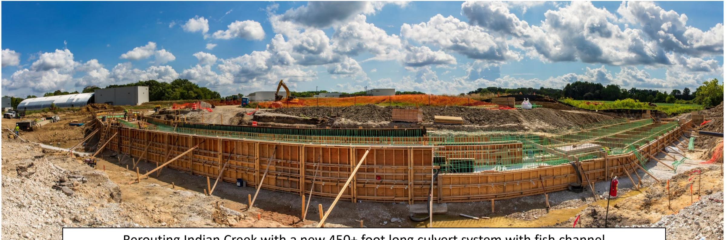
Rerouting Indian Creek with a new 450+ foot long culvert system with fish channel
