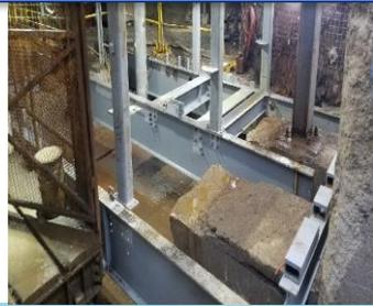
Installing sump at 5000' level
