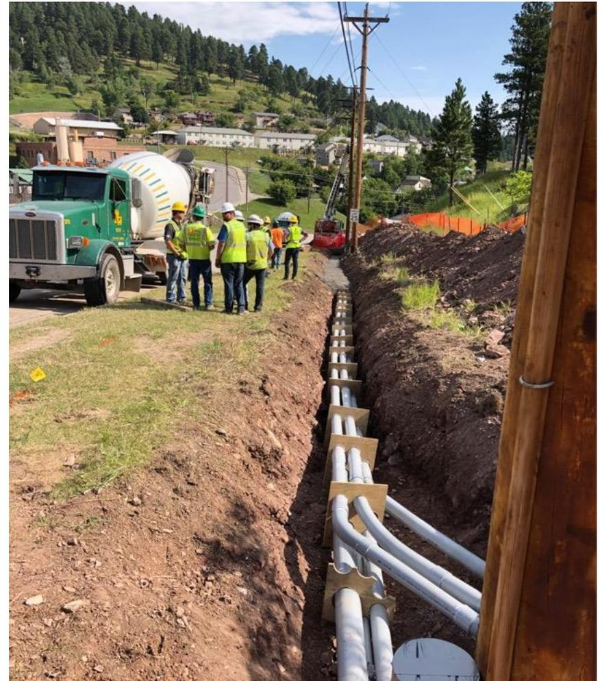
Rerouting power underground so elevated conveyor can cross state highway
