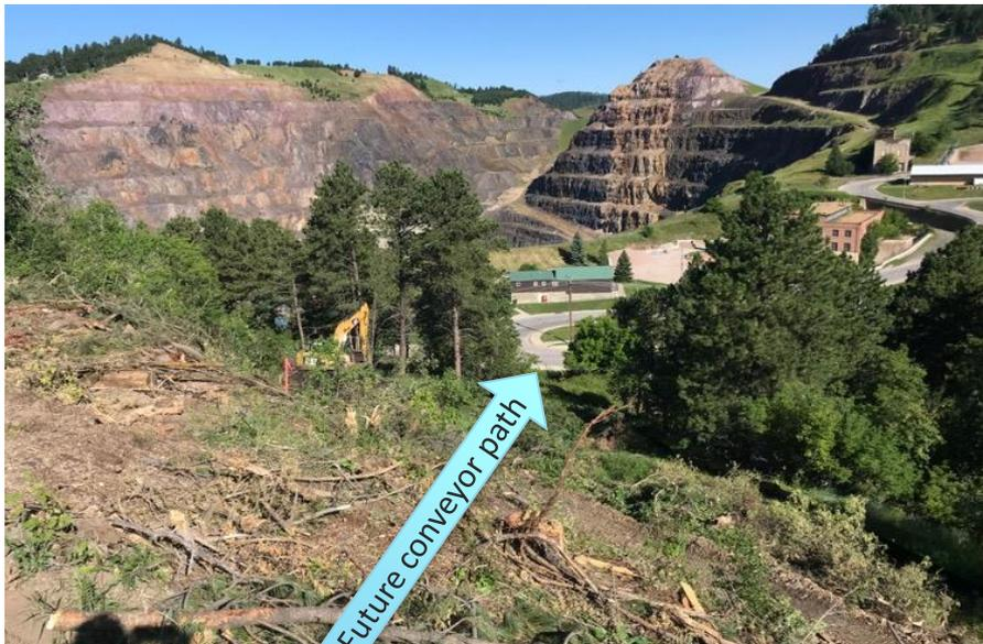
Clearing path for elevated conveyor to open cut
