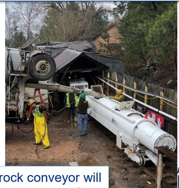
Refurbishing the 2400' long tramway that the 4100' rock conveyor will be installed in to move rock to the open cut in downtown Lead, SD
