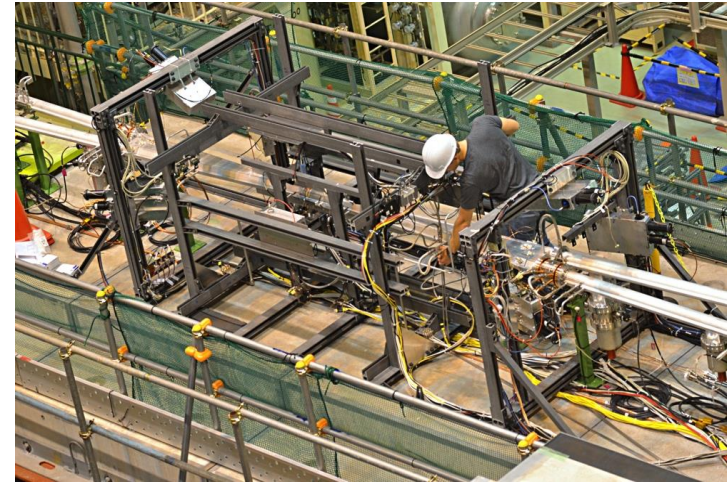
Accelerator background commissioning detector is installed and working at the IP
