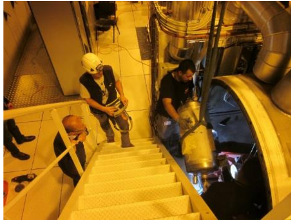
Earlier removal of 80 K adsorber
