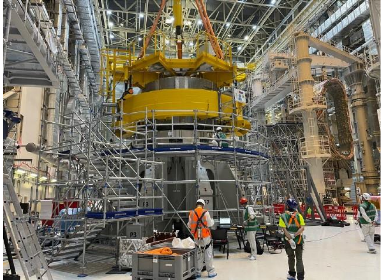
Central solenoid module assembly progressing at the ITER site
