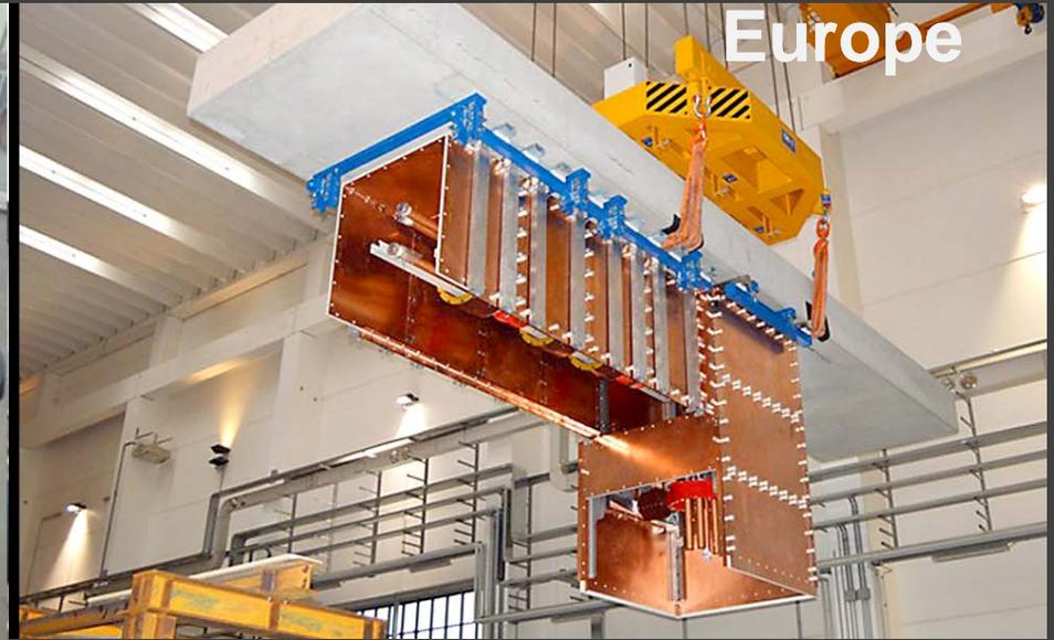
Part of the 35m transmission line connected to the SPIDER vessel at the Neutral Beam Testing Facility (NBTF) site in Padua, Italy.
