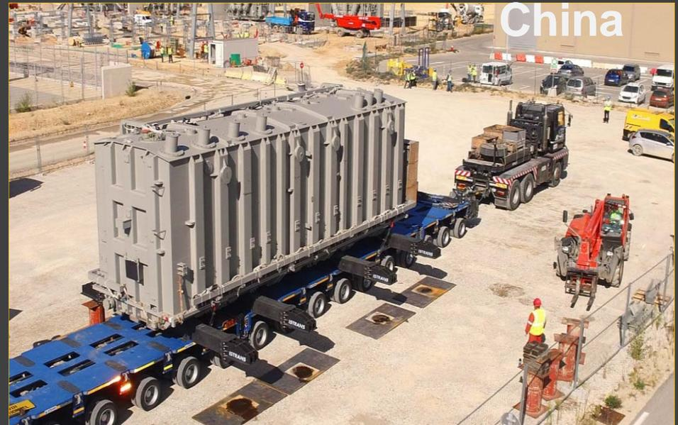
The first of three power transformers for the pulsed electrical network is being equipped on site.
