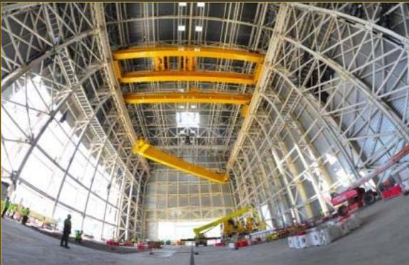
◀ On 22 June, the 4 beams and 2 of 4 trolleys (100 t.) are installed.
