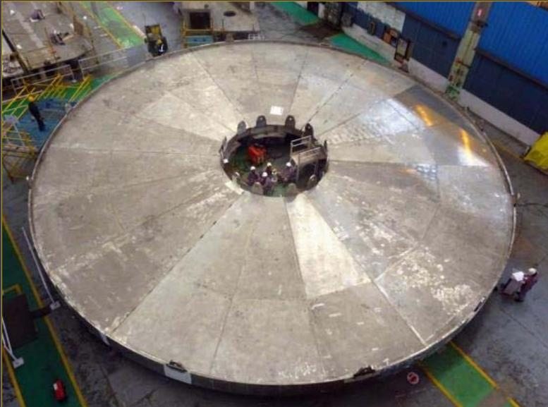
India is responsible for fabrication and assembly of the 30 x 30 meter ITER cryostat. The base plates for Tier 1 & 2 have been delivered to ITER.
