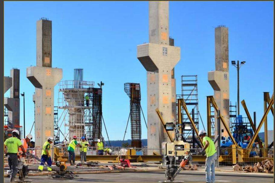
Foundation works and column construction are ongoing on what will be the largest single platform cryoplant in the world. The ITER Cryoplant will distribute liquid helium and nitrogen to various machine components (superconducting magnets, thermal shield, cryopumps, etc.).
