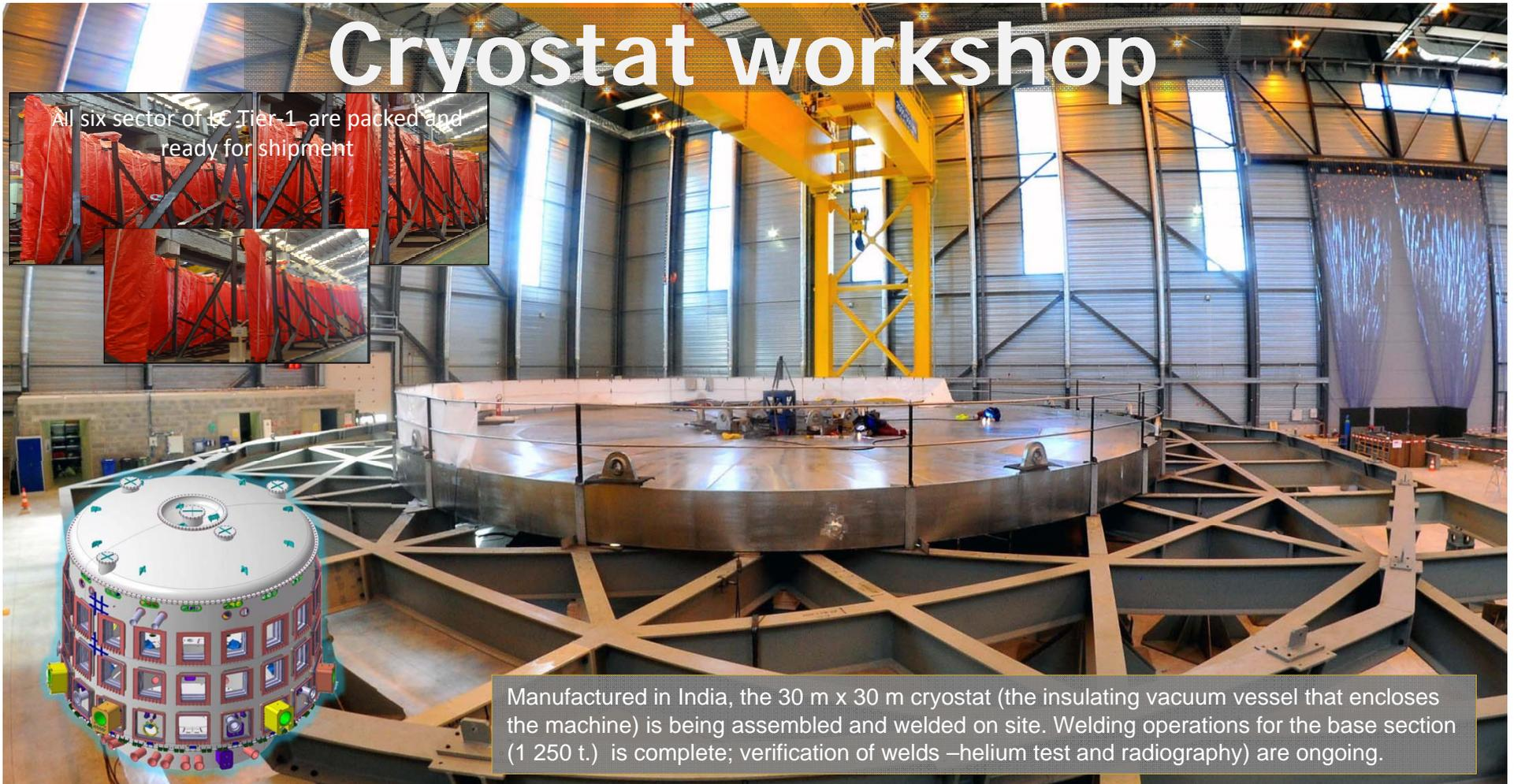
Manufactured in India, the 30 m x 30 m cryostat (the insulating vacuum vessel that encloses the machine) is being assembled and welded on site. Welding operations for the base section (1 250 t.) is complete; verification of welds –helium test and radiography) are ongoing.
