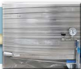
1: Conductor receiving inspection
