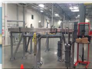
3: Joints & Terminals Preparation
