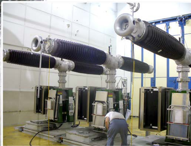
One of four sets of 400kV, 3-phase HV circuit breakers undergoing factory acceptance test at Alstom SAS, Villeurbanne, France
