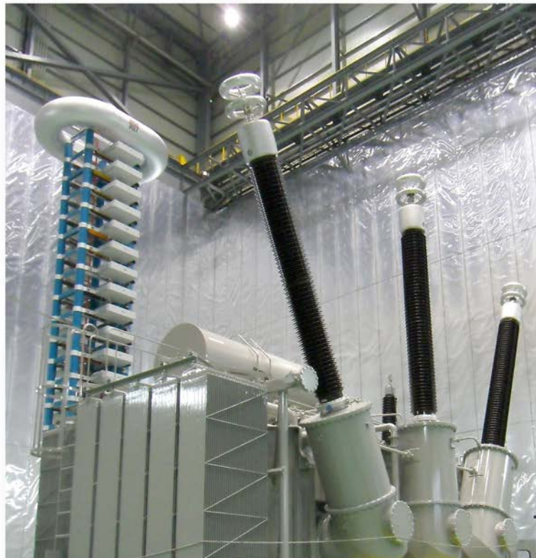
First of four HV substation transformer units undergoing factory acceptance tests at the Hyundai Heavy Industries factory in Ulsan, Korea
