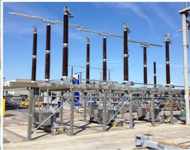
One of four 400kV, 3-phase HV disconnect switches undergoing factory acceptance tests of the Alstom SpA factory in Noventa di Piave, Italy
