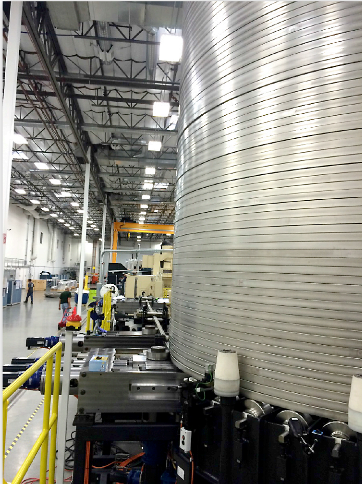
Conductor routed from de-spooler
