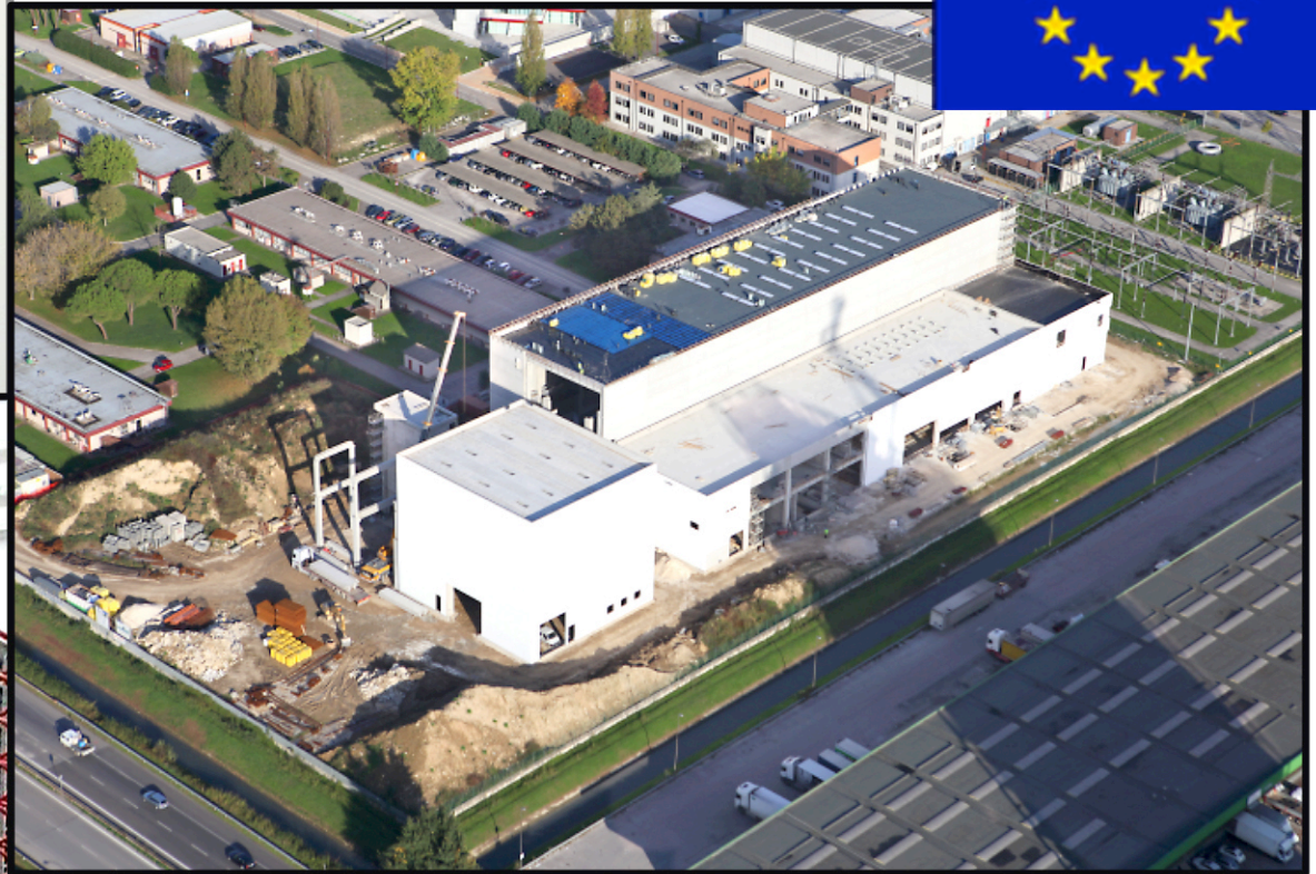
Neutral beam injector test facility in Padova, Italy
