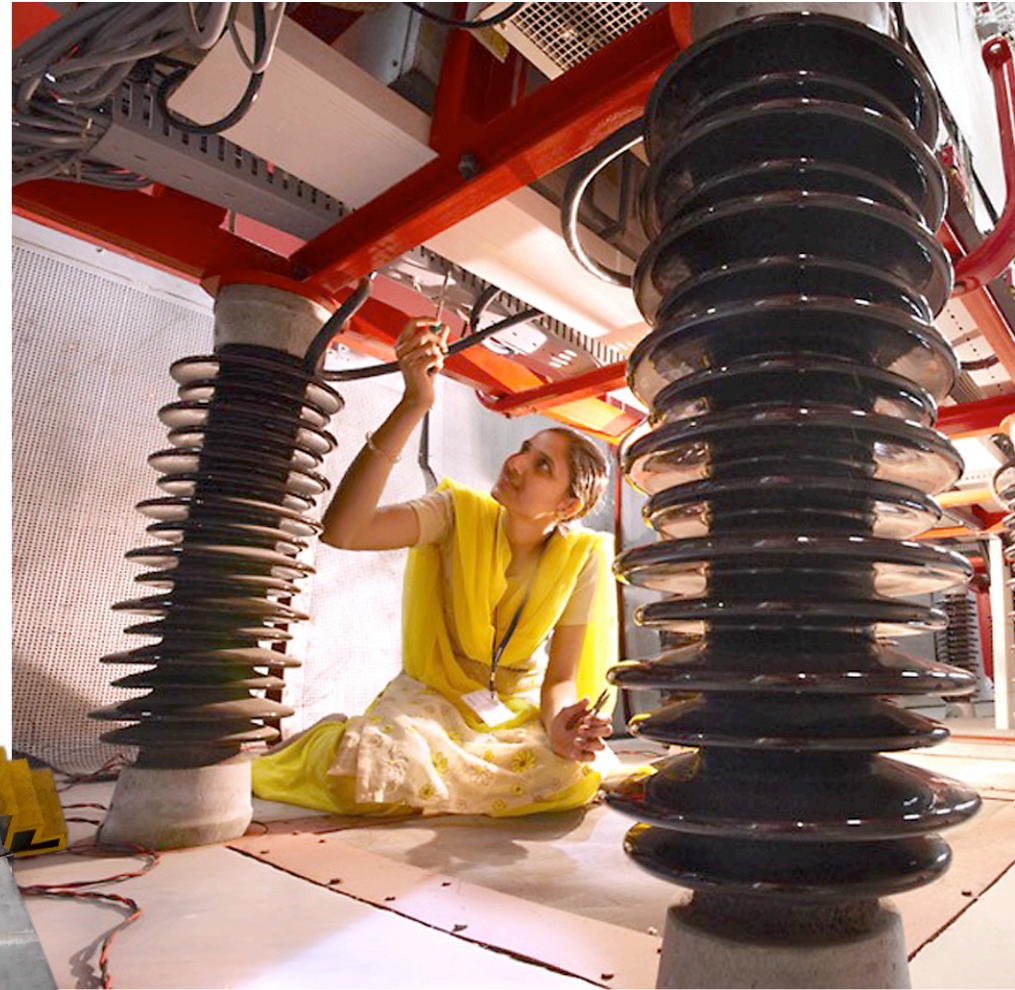
High voltage power supply for Diagnostic Neutral Beam. Photo: IN DA
