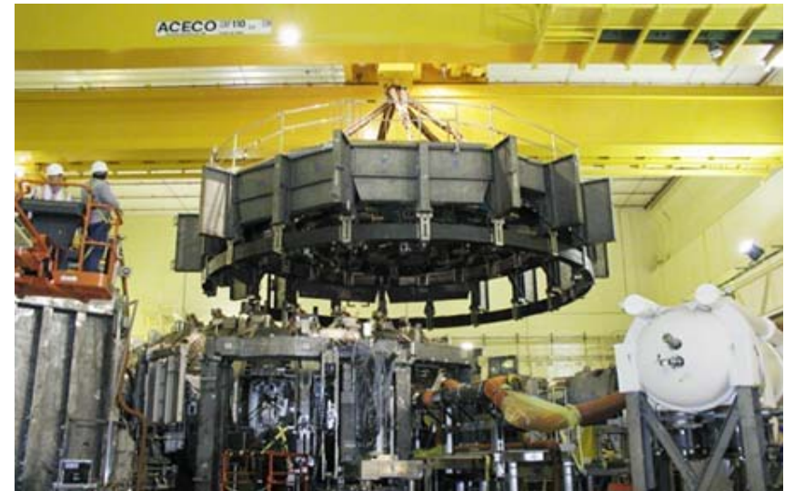
Removal of the TFTR Umbrella Structure
