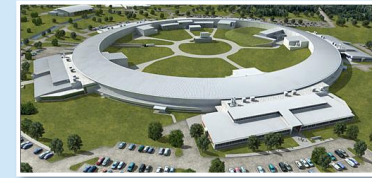
National Synchrotron Light Source-II (BNL)
