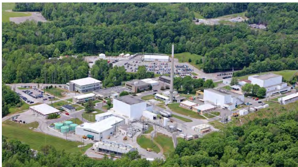
FIGURE A1.2. ORNL’s High Flux Isotope Reactor (HFIR) campus including the Radiochemical Engineering Development Center (REDC)
