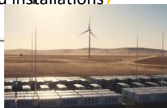
Southwest event: Grid installations
