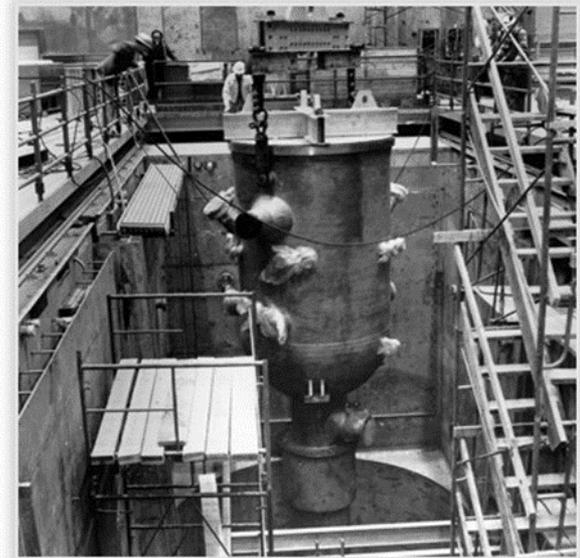
The HFIR pressure vessel built by the former Allis-Chalmers Manufacturing Company was installed in April 1964 and has continued to operate reliably for more than 55 years.
