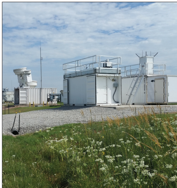
Fig. 15. Radar Row. In 2016, the ARM Southern Great Plains site reconfiguration took another step toward completion with the Raman lidar's reinstallation near the scanning radars, commonly referred to as ARM's radar row. [Courtesy ARM User Facility]
