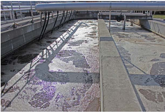
Wastewater treatment plant in Klosterneuburg, Austria
