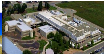
Combustion Research Facility
