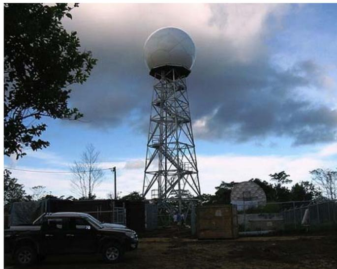
cm-wavelength radars focused on precipitation and storm dynamics are deployed at Oklahoma (X and C-band) Barrow (X-band), and Manus (C-band).
