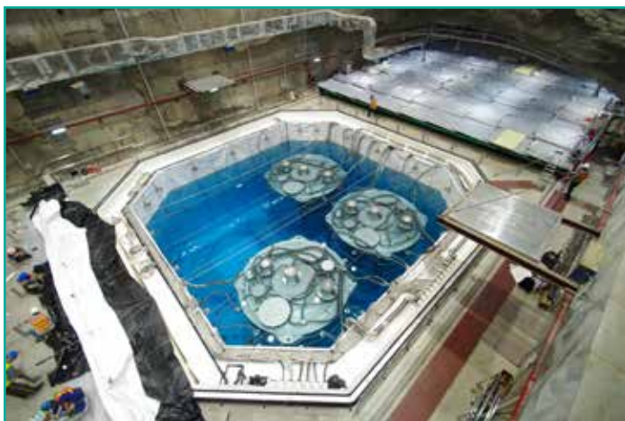
The Far Hall (EH3) water pool with 3 Anti-neutrino detectors in place before the pool cover is installed.
