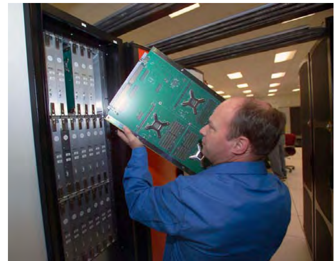
Replacing an upgraded board
