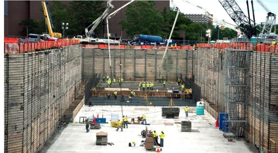
Workers placing 1,400 cubic yards of concrete in the first structural concrete placement in July for the linear accelerator tunnel.
