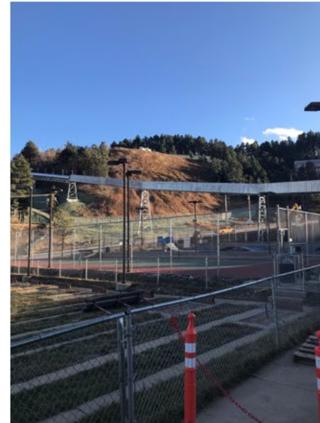
Rock Conveyor crossing road and public spaces
