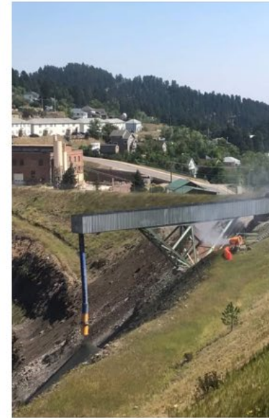
Depositing Rock in Open Cut
