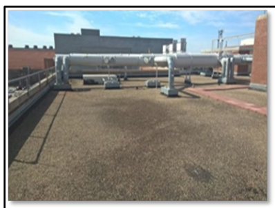
Spedding Hall Existing Built-Up Roof (circa 1985)
