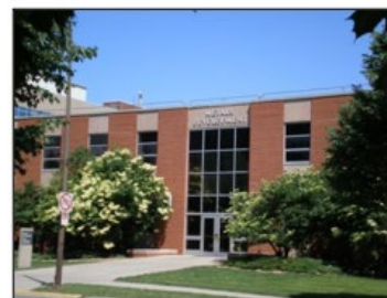
Metals Development Building (1961)
