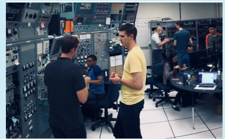
Tandem Control Room at TUNL [S71]
